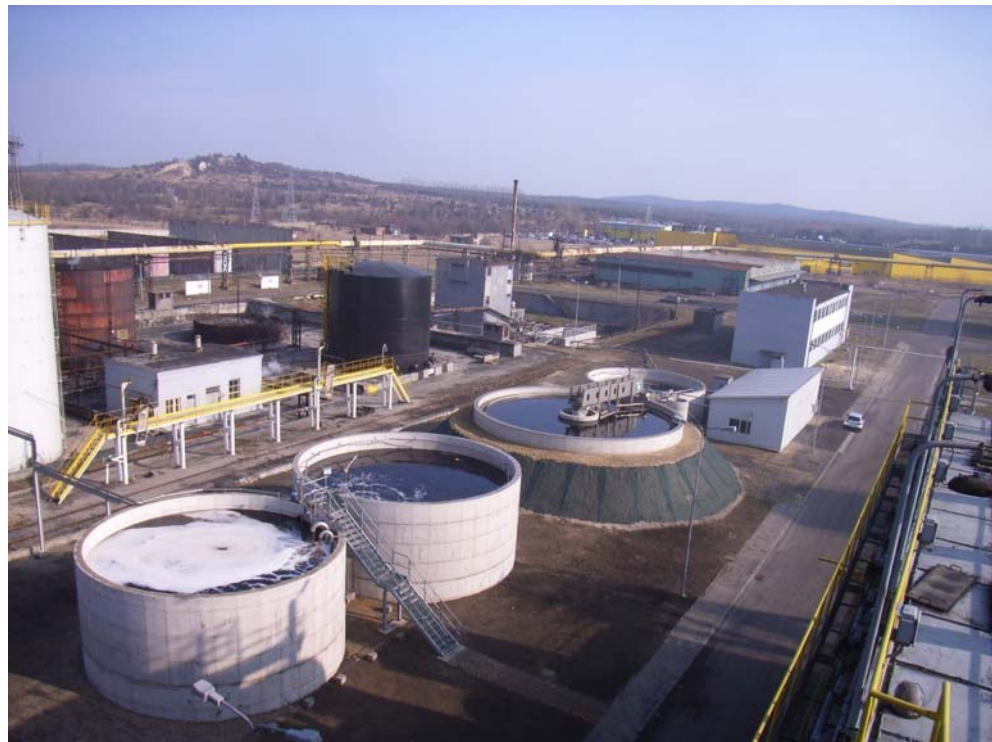
Coke oven wastewater treatment plant with Mutag BioChip™ in Poland
