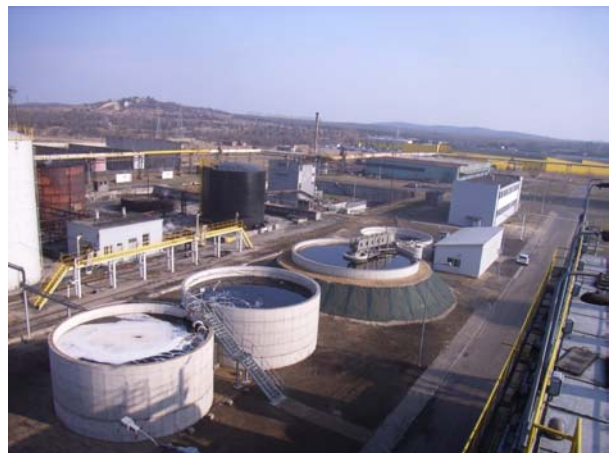
Fig. 2: Coke oven wastewater treatment plant with Mutag BioChip™ in Poland
