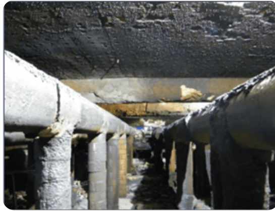
Fig 5: Interior of a hot strip mill reheat furnace.
